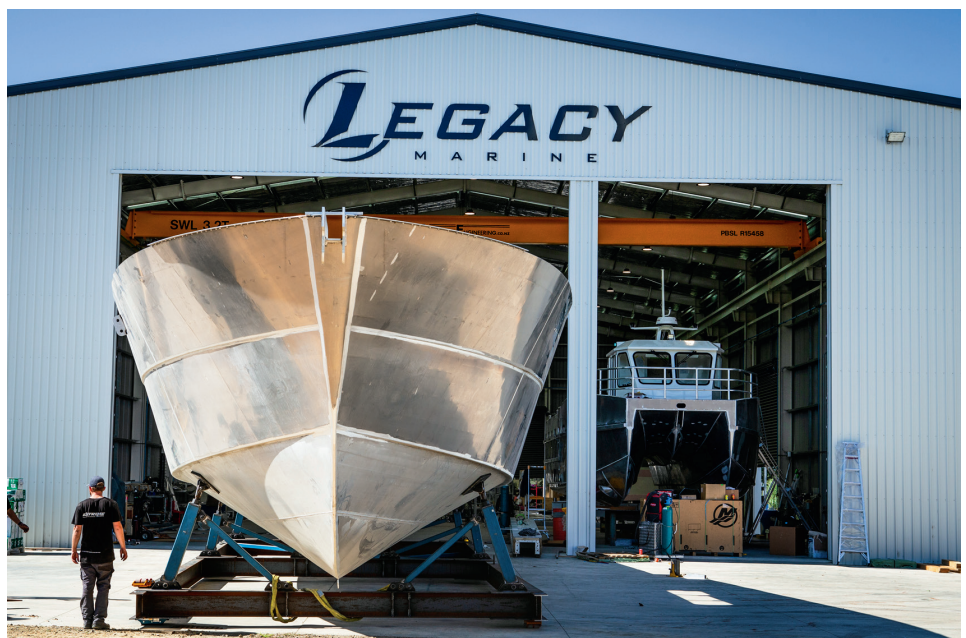
Legacy Marine has just turned the hull of its first sportfisher, the largest in its range at 21.5m.
